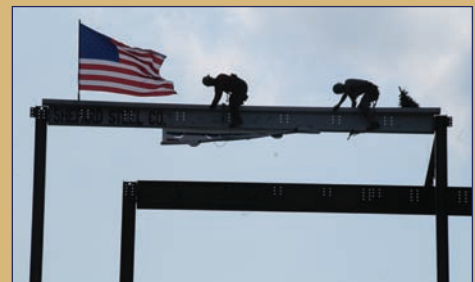
Workers place the last steel beam into position
